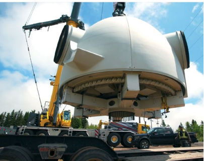
The nacelle of a decommissioned turbine is lowered to the ground. Fitzpatrick Mountain Wind, Nova Scotia.
